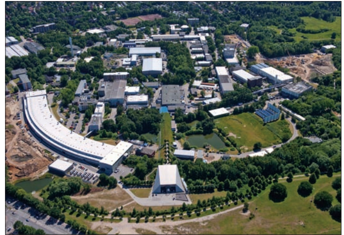
Bird's eye view of the DESY research centre in Hamburg. The 260 m-long FLASH free-electron laser with its experimental hall can be seen in the foreground. On the left of it is the large new experimental hall of the PETRA III synchrotron radiation source. The DESY site is encompassed by the 2.3 km PETRA III storage ring. On the upper right side of the picture, near the former HERA refrigeration hall, is the construction site of the injector complex for the European X-ray laser XFEL, a 3.4 km-long free-electron laser facility that will run from the DESY site in a north-western direction towards the town of Schenefeld. The halls of the 300 m-circumference DORIS III storage ring can be seen between the PETRA III experimental hall and the beginning of the FLASH linear accelerator. (Courtesy Reimo Schaaf, Schönwalde.)
